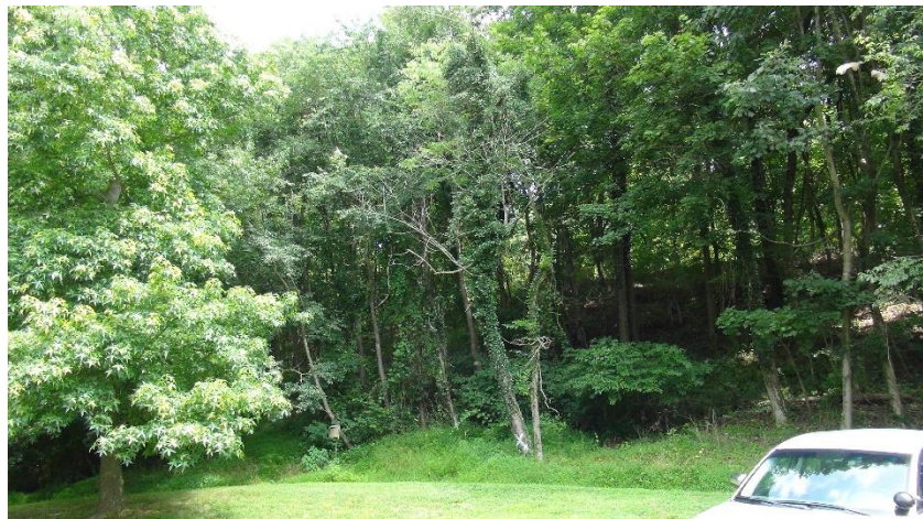
We have several dead and dying trees that require removal.
